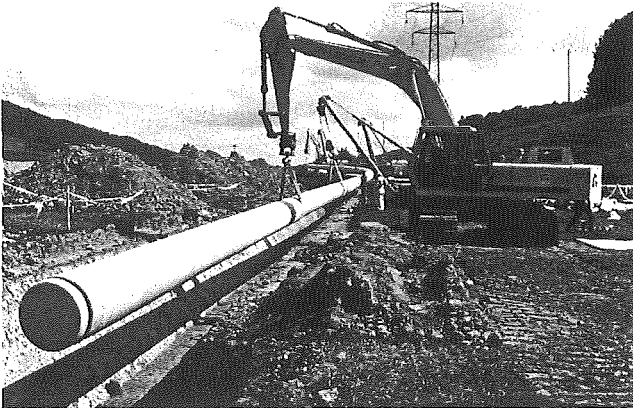
Fig. 1 Placement of pipeline tubes
